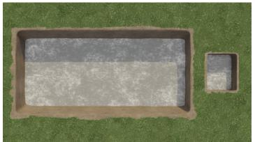
The concrete slab should also be prepared for the filter room. There is no need to reinforce the slab
